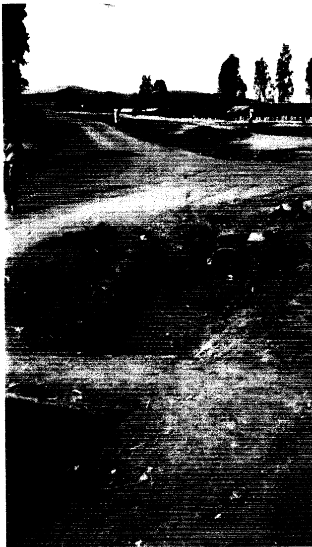
JUNCTION SERVICE ROAD WITH NYARUTARAMA ROAD HIGH TENSION LINE SERVING AREA. POOR ROAD SURFACE AND DRAINAGE
